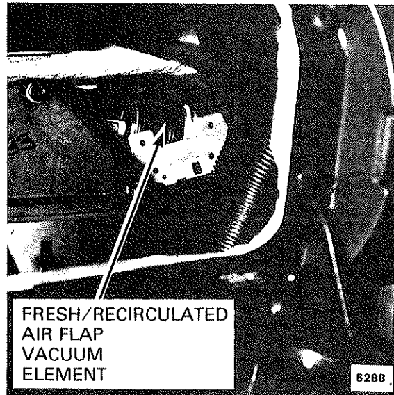
Figure 4 - Behind Glove Box
